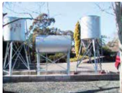
Bunded fuel storage
